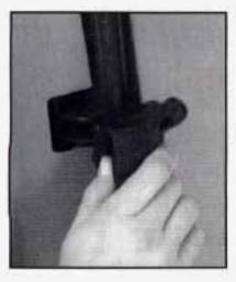
To open, pull the latch forward to release it, then swing the window outward. Press the center of the latch to secure the window in the open position.
